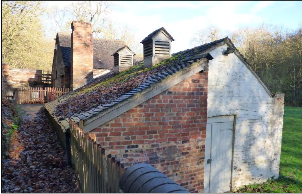
Figure 8: Roof top vents and chimney stack identify the drying kiln at Mosty Lea Mill
