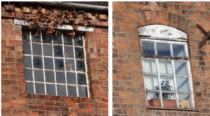
Figures 17 & 18: Multipane window at Stone Mill with dentillation to eaves above, and replacement window with simple segmental arched header.
