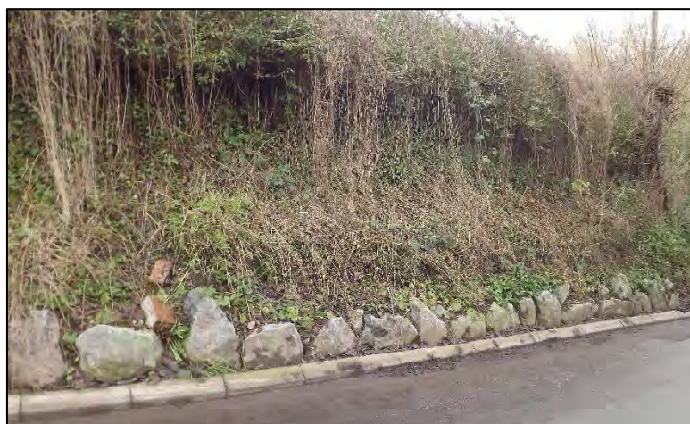
Figure 78: Insertion of standard concrete kerbing in place of soft verge
