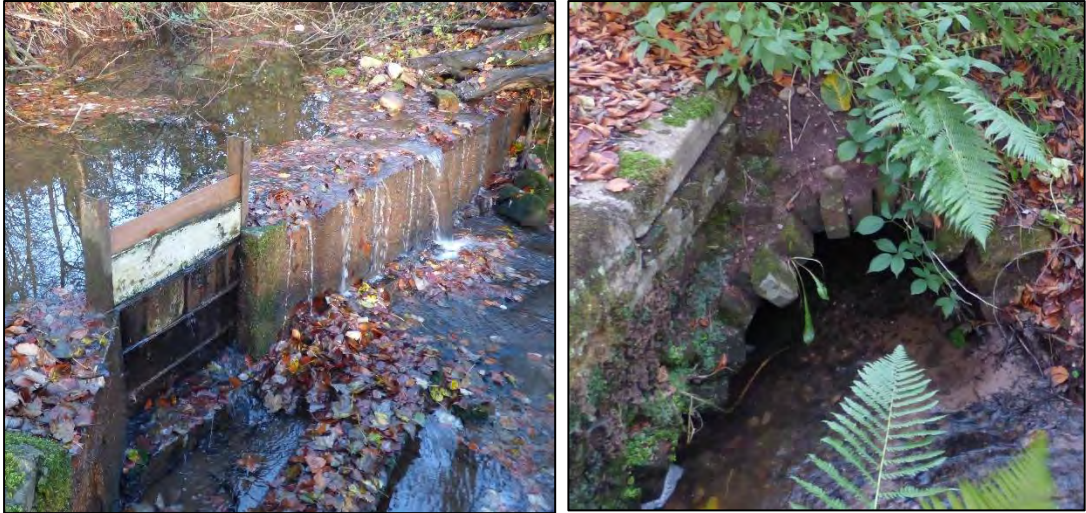
Figures 11 & 12: Sluice gate and weir between Wetmore and Mosty Lea Mills, and brick-lined culvert taking the stream under Mill Lane from Splashy Mill to the former Ochre Mill site
