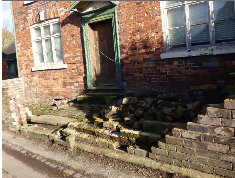
Figure 76: Damaged wall at Boulton's Offices, Moddershall
