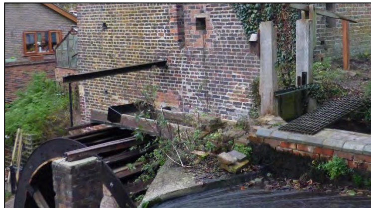
Figure13: Wooden laundry and sluice gate at the overshot wheel of Splashy Mill
