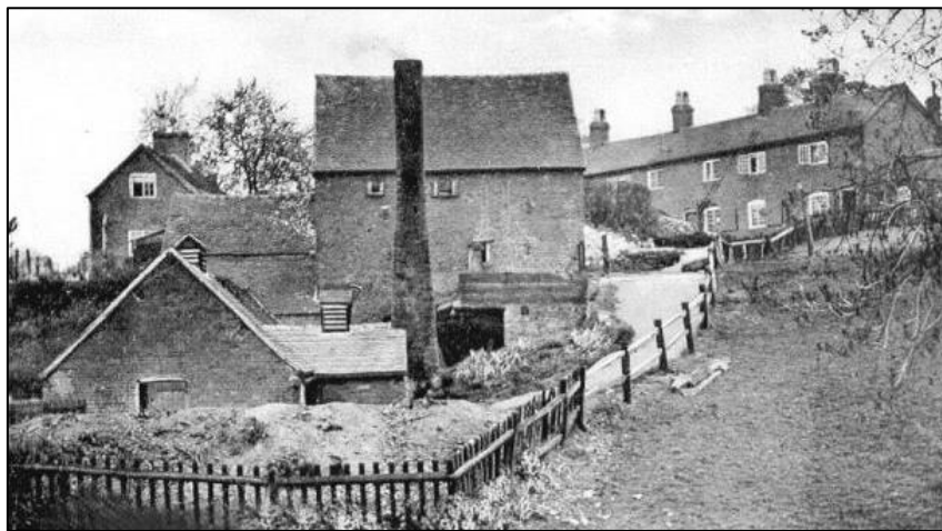
Figure 14: Exposed brick elevations at Hayes Mill, Hayes House, and Millbank Cottages, c.1900, now all painted or rendered.
