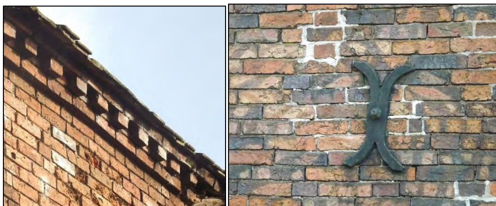
Figure 55 & 56: Dentilled eaves and burnt brick in Flemish bond with traditional cast iron tie bar bracket
