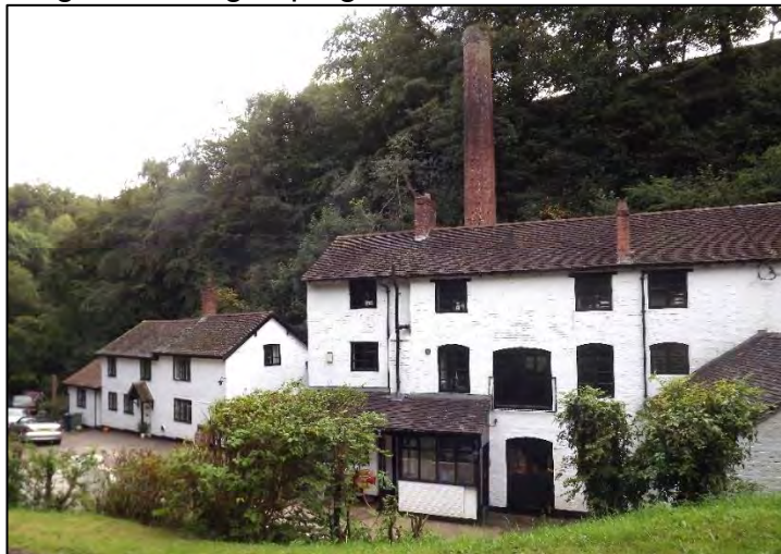
Figure 32: Ivy Mill, with cottages to the left and industrial mill to the right.
