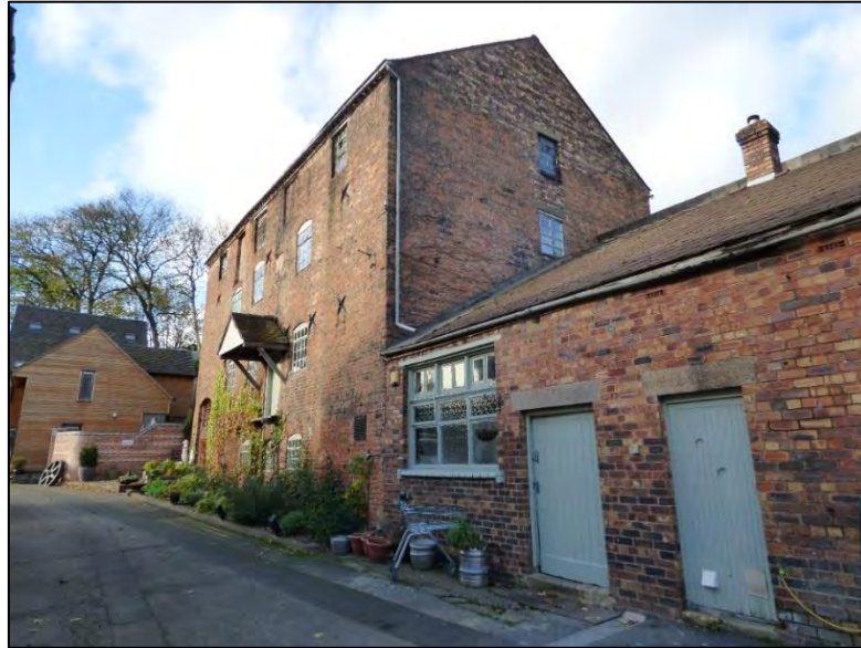
Figure 40: Stone Mill, now in use as a restaurant
