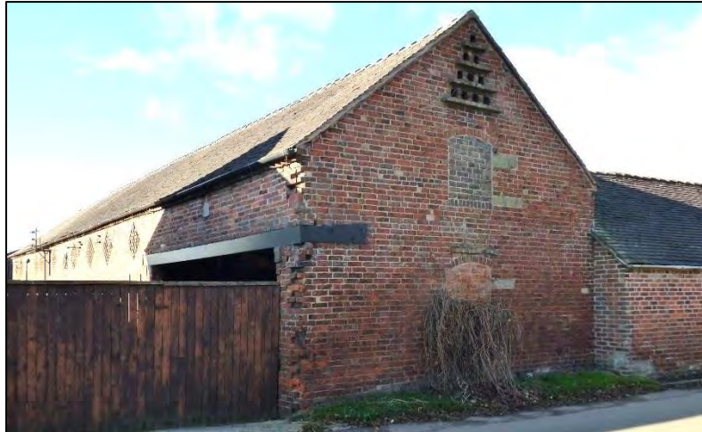
Figure 68: Barn at Moss Rose Farm with blocked up pitching door and openings for pigeon loft above.
